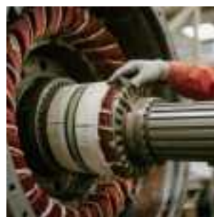
Generator Stator Inspection
